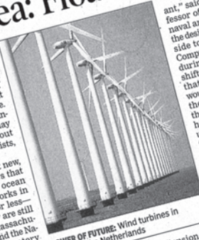
POWER OF FUTURE: Wind turbines in Dronten, the Netherlands
