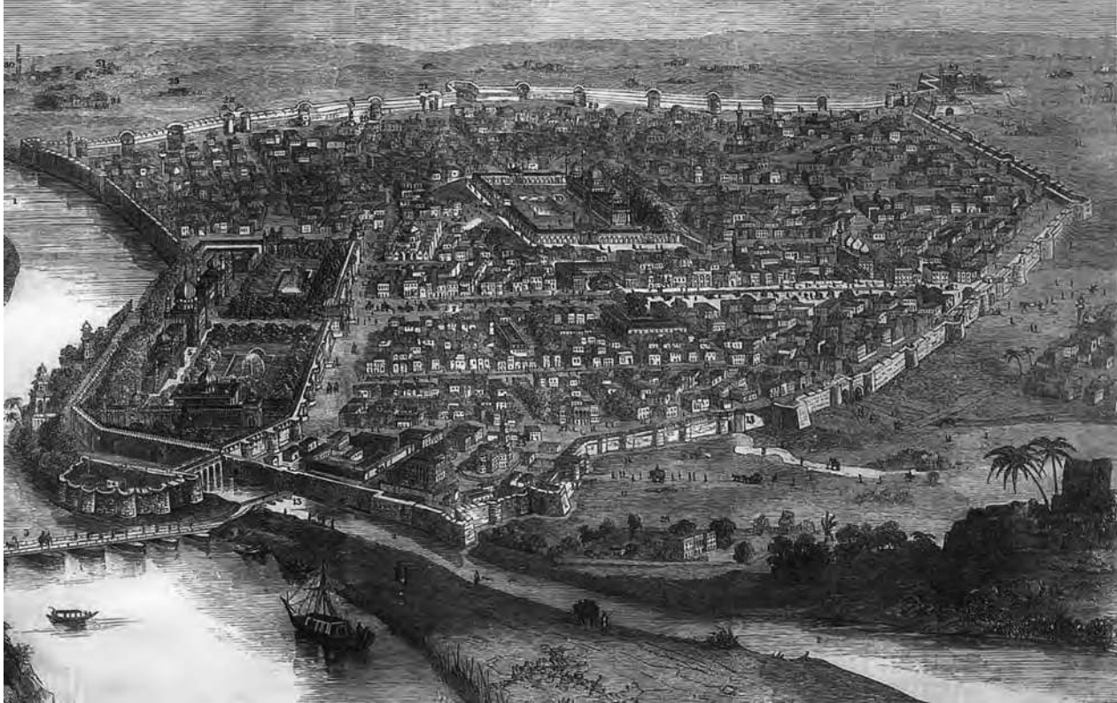
Fig. 3 – Image of Shahjahanabad in the mid-nineteenth century, The Illustrated London News , 16 January 1858 You can see the Red Fort on the left. Notice the walls that surround the city. Through the centre runs the main road of Chandni Chowk. Note also the river Jamuna is flowing near the Red Fort. Today it has shifted course. The place where the boat is about to embark is now known as Daryaganj ( darya means river, ganj means market)
