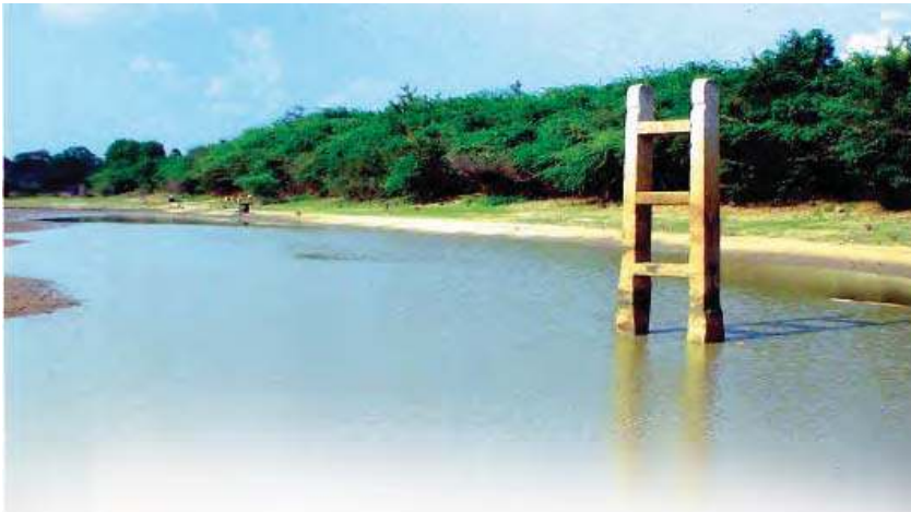
Fig. 5 A ninth century sluiceway in Tamil Nadu. It regulated the outflow of water from a tank into the channels that irrigated the fields.
