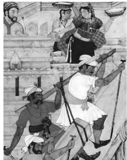
Fig. 8.8 b Women carrying loads Migrant women from neighbouring villages often worked at such construction sites.
