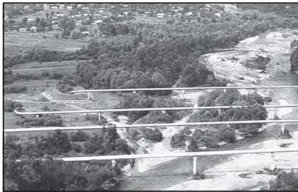
Fig. 8.17: Pipelines transporting natural gas in Ukraine
