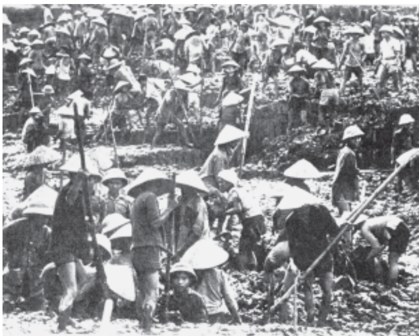
Fig. 15 – Rebuilding damaged roads. Roads damaged by bombs were quickly rebuilt.
