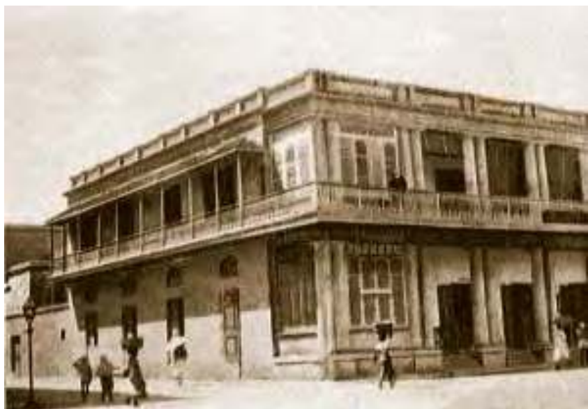
Fig. 22 – The first office of the Madras Chamber of Commerce. By the late nineteenth century merchants in different regions began meeting and forming Chambers of Commerce to regulate business and decide on issues of collective concern.
