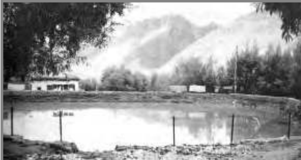
A kul leads to a circular village tank, as the above in the Kaza village, from which water is released as and when required.
